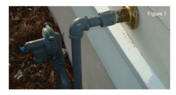
flange must be completed using black iron pipe and fittings (See Figure 1).
